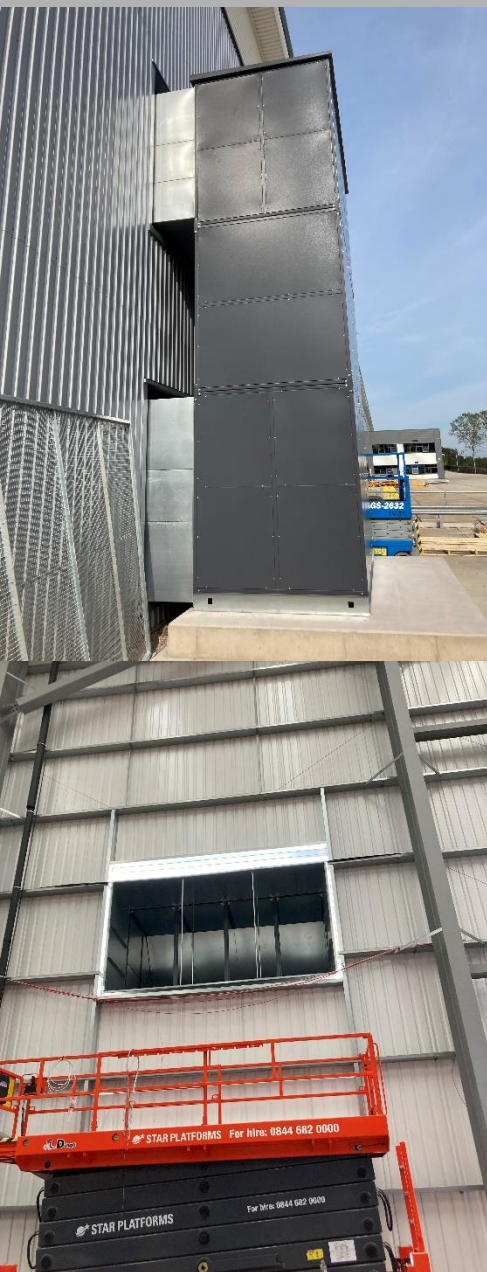
Powrmatic TE61 during installation
